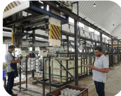
Electro Plating Plant Automatic & Manual
